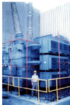
PJM Public Service Step Up Transformer Severe internal damage caused by the space storm of 13 March, 1989.
