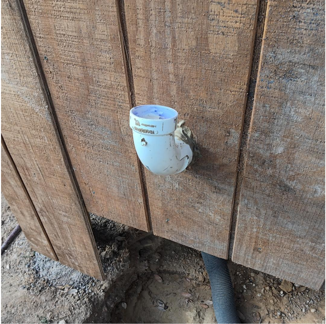
After the T-111 siding is up, ran a 2 inch vent pipe outside, then a 90 degree elbow up.
